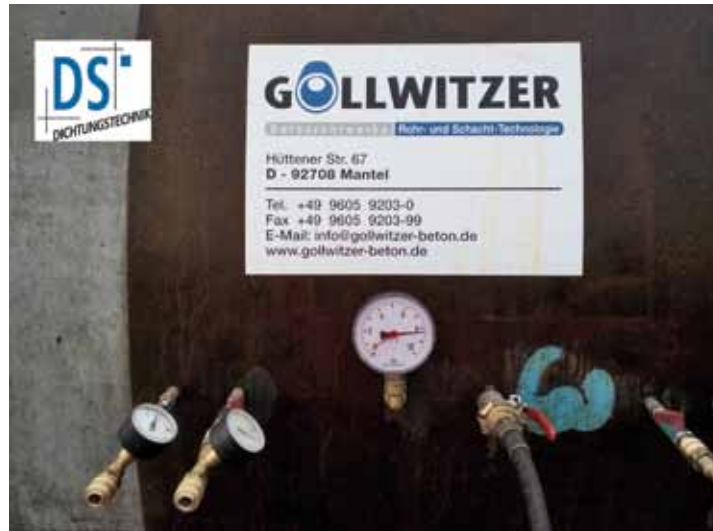
The external chamber pressure, simulated by means of a steel sleeve above the two reinforced-concrete pipes, amounted to a maximum of 8.25 bar and could be kept for 60 minutes without pressure loss
